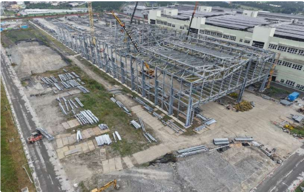
Maintenance Workshop Construction Area
