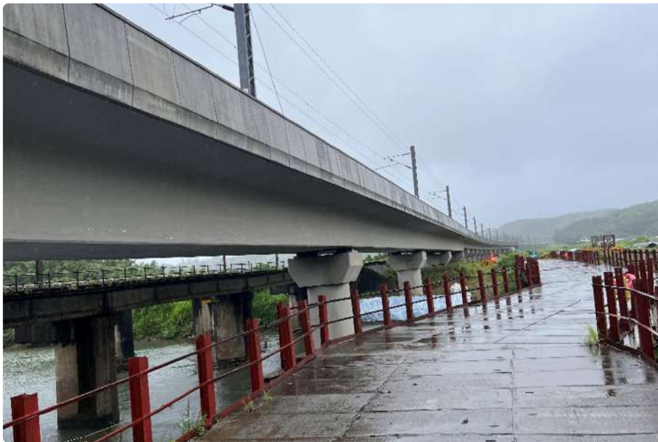
Reconstruction of the No.3 Shuangxi Bridge and Xinshe Bridge—Upward View of the Bridge from Below
