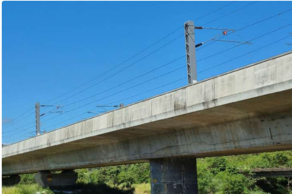
Reconstruction of the No.1 and No.2 Shuangxi Bridges—Bridge Underside
