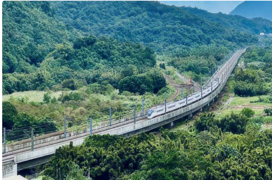
Actual Site View After Track Diversion—No.1 and No.2 Shuangxi Bridges
