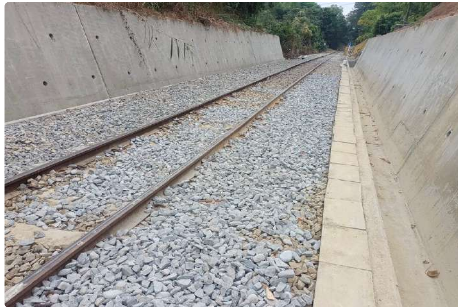
Slope Improvement to Strengthen Structural Safety
