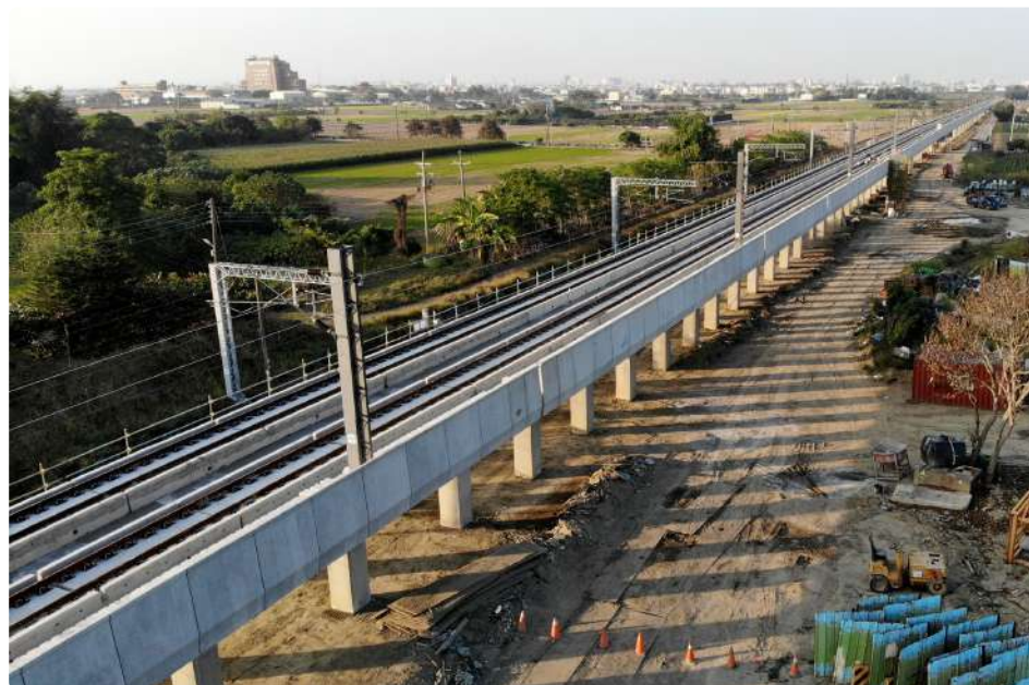
Reconstruction of the Wencuobu Creek Bridge
