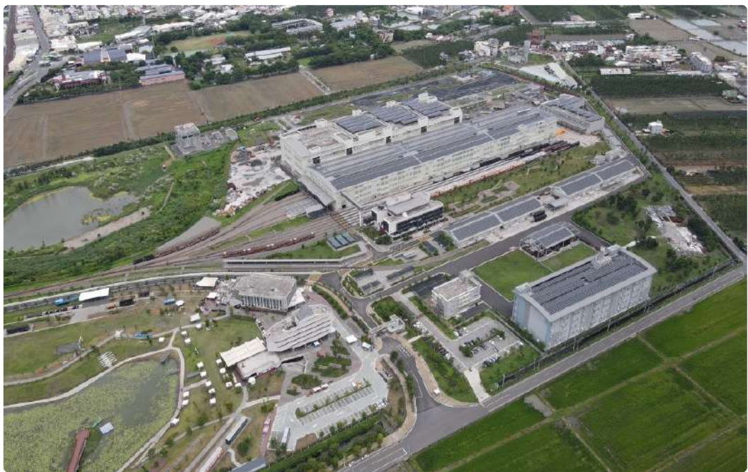
Chaozhou Rolling Stock Depot—On-Site View
