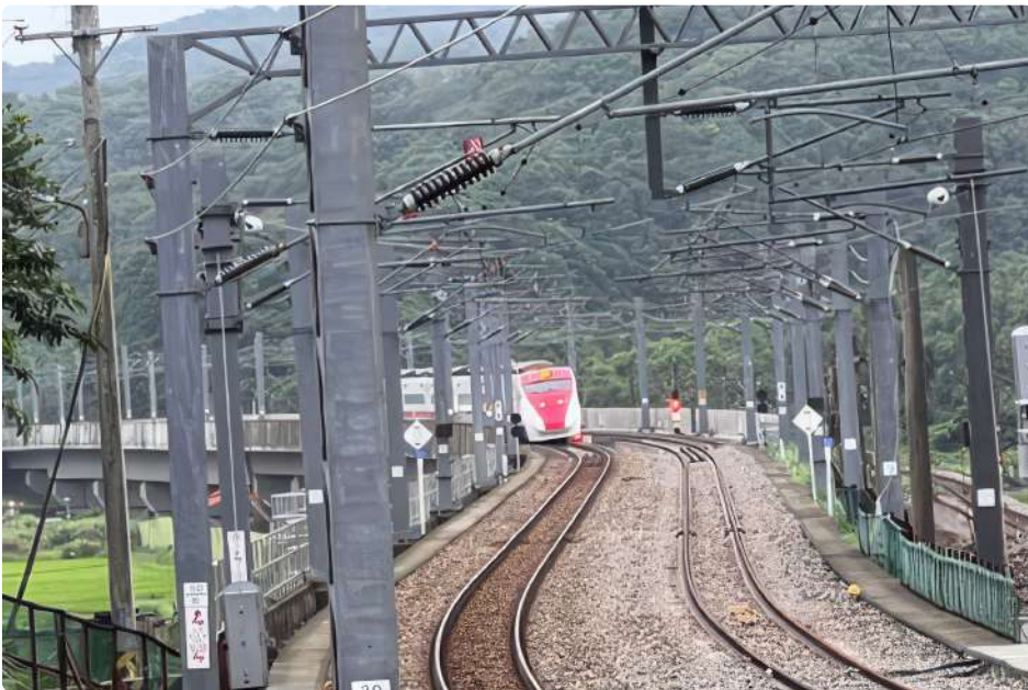
Reconstruction of the No.3 Shuangxi Bridge and Xinshe Bridge—Section where Puyuma trains operate
