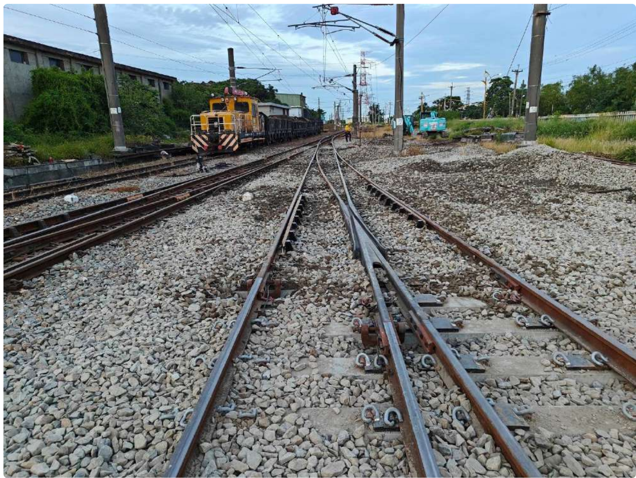
Turnout Renewal at Tongxiao Station
