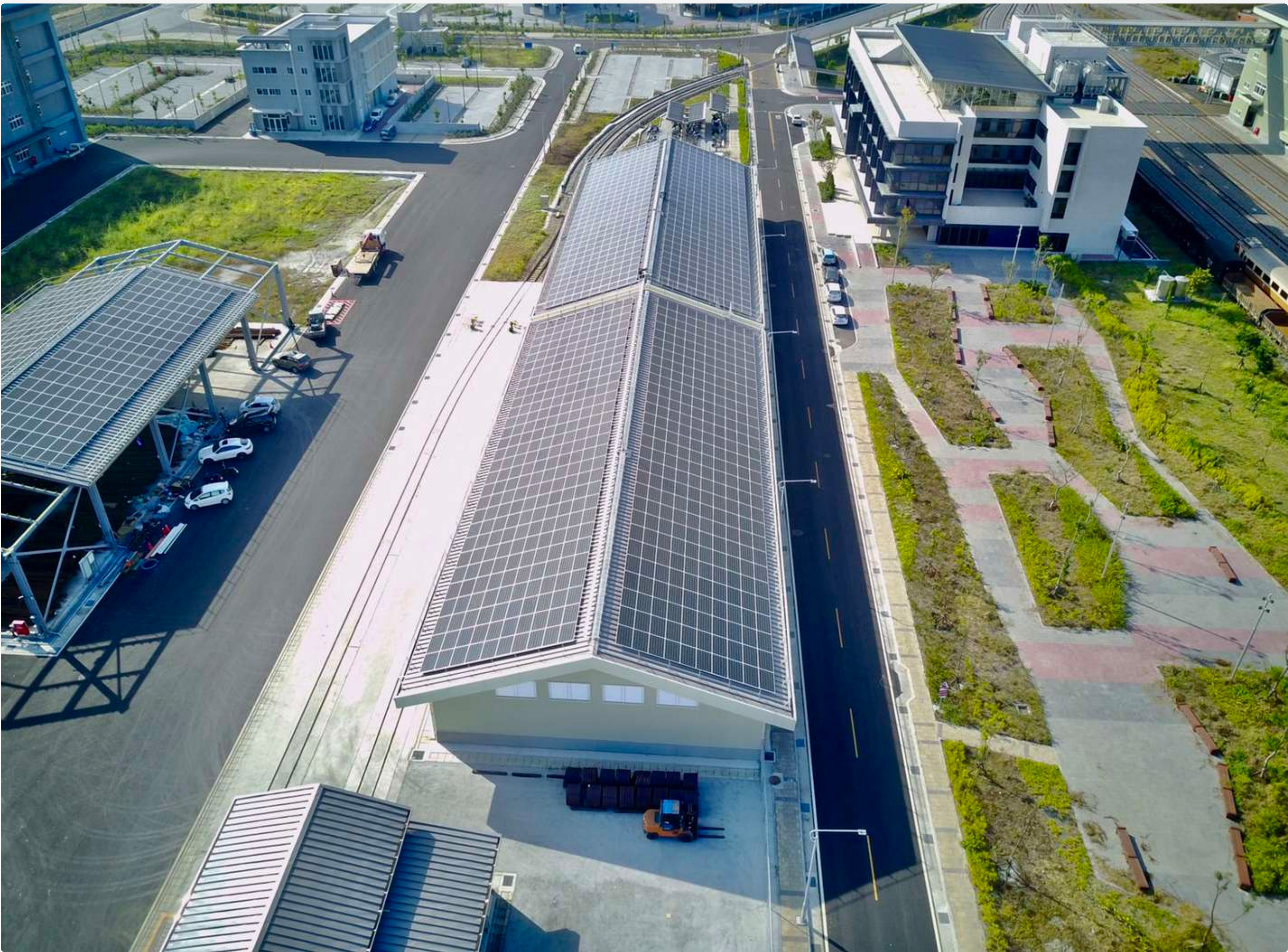
Rooftop Solar Photovoltaic Installation at the Chaozhou Rolling Stock Base
