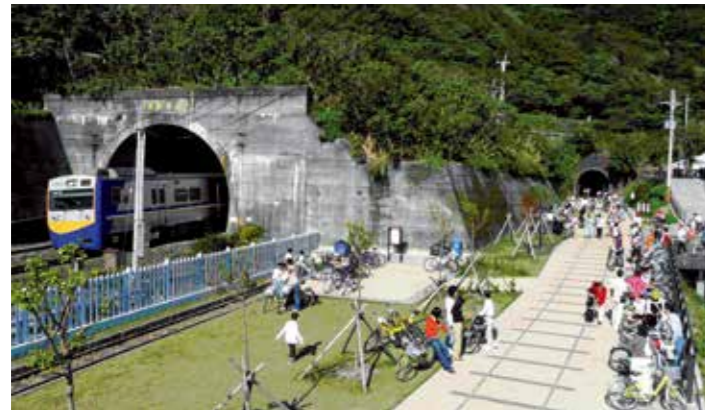
台鐵局無償提供舊草嶺隧道，為民眾打造低碳樂活的自行車道。 The TRA promotes low-carbon lifestyles by providing a cycling trail through Caoling Tunnel.
