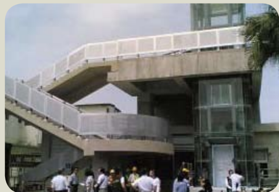
完成彰化跨站天橋 Completed elevated bridge at Changhua station
