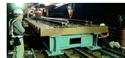
New beam installation
