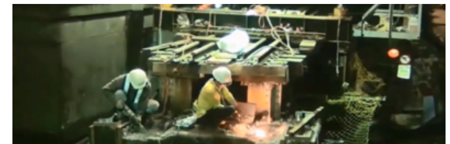
Removal of original pier surface
