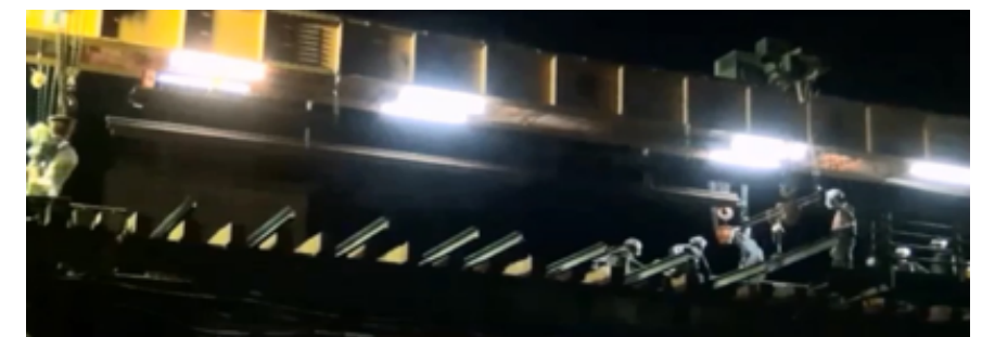
C channel pedestrian path installation
