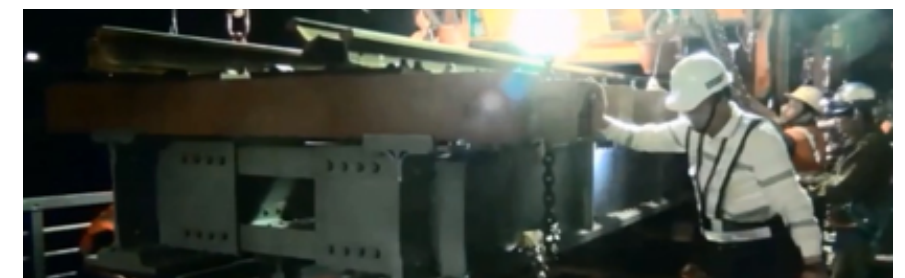
Entry of the new beam, level hoist with a U-shape ring
