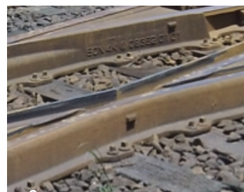
Serious crush at the crossing nose.
