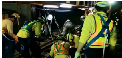
Track fastener installation
