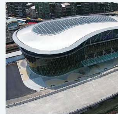
屋頂以太陽能系統設計，強化車站節能。 Roof is designed with solar energy system to support station power need.
