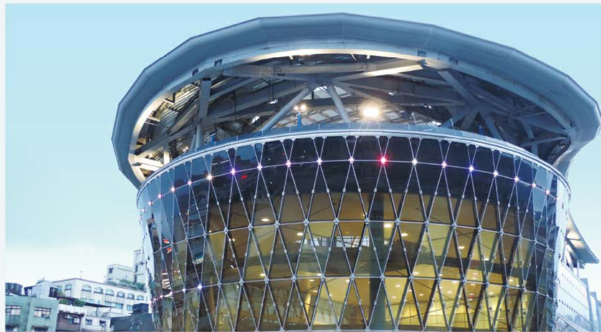
南站外牆以玻璃帷幕搭配金屬板，營造空間虛實變化。 Wall of south entrance is made of glass together with metal plate
