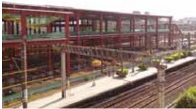
▲ 桃園臨時站工程 Construction of a temporary platform for Taoyuan Station
