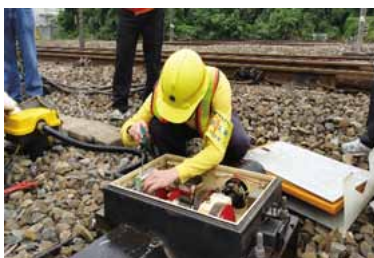
▲ 電動轉轍器調校檢測 Electric switch adjustment and examination
