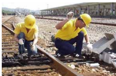
▲ 電動轉轍器調校檢測 Electric switch adjustment and examination
