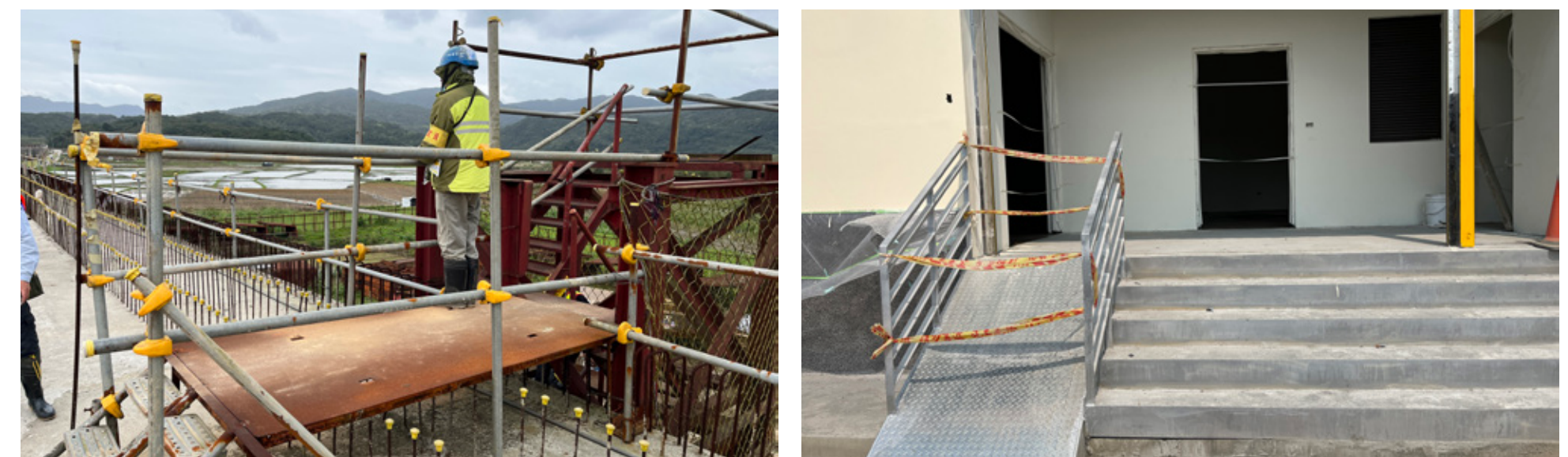
Project supervision without prior notice was implemented for construction in progress
