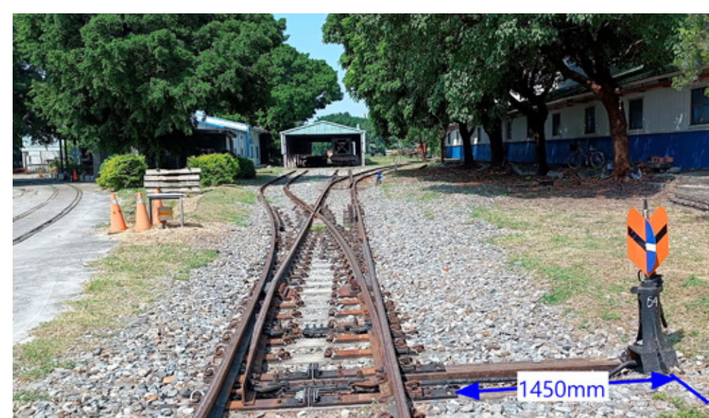
Image ⑤ Articulated left switch 50 kg-N #8 articulated left switch, the distance between the medium-sized marker-type switch and the plate is 1,450 mm
