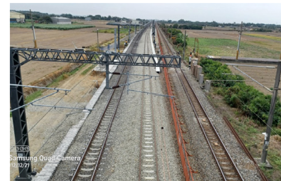
Wencuobuxi Bridge reconstruction project
