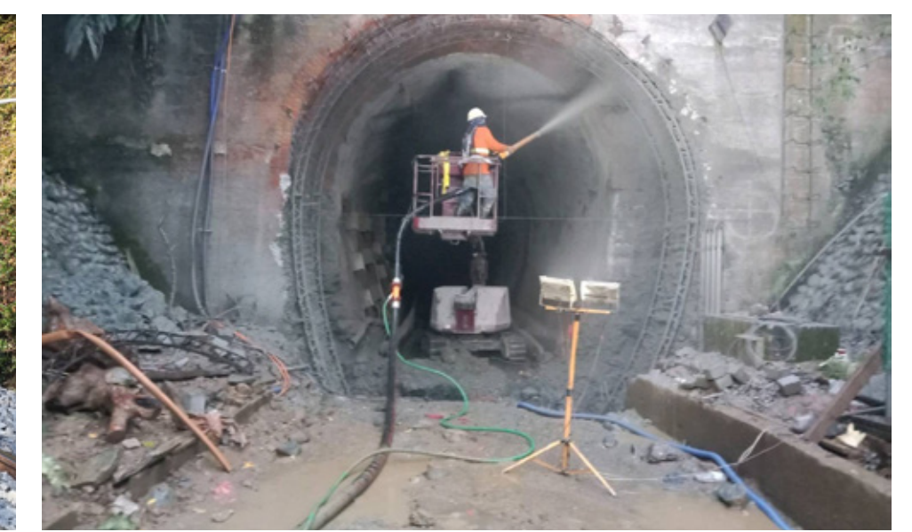
Tunnel and slope improvement turnkey project (shotcrete pouring)
