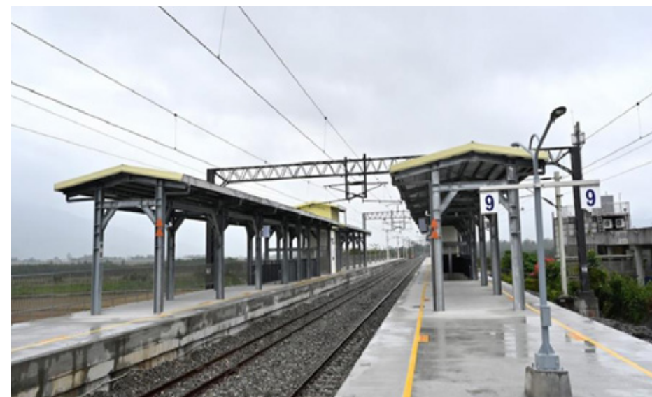
Platform elevation was completed at Dongli Station
