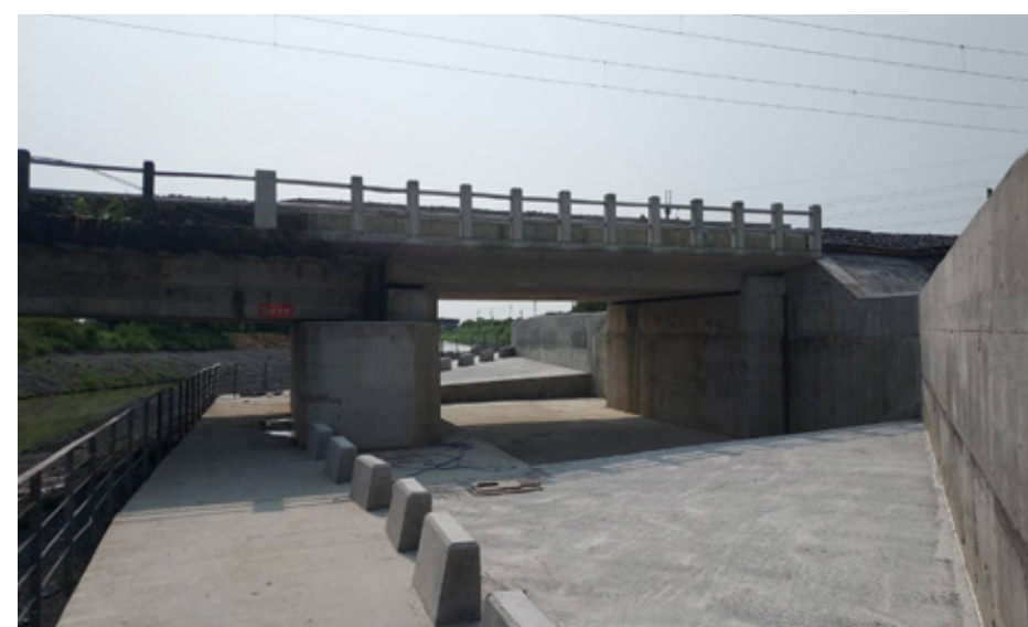
Xiaqijie Bridge reconstruction project (south side)
