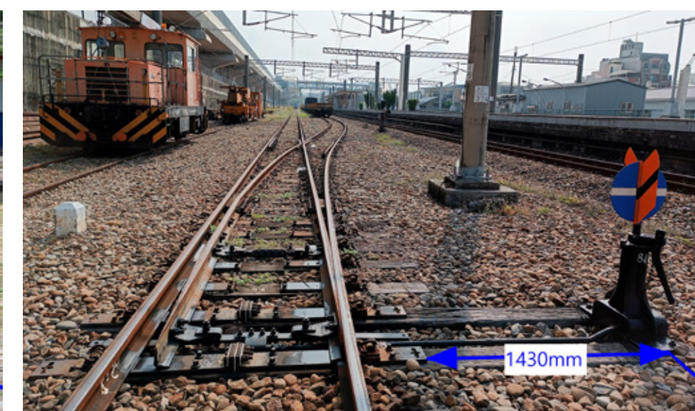
Image ④ Articulated right switch 50 kg-N #8 articulated right switch, the distance between the medium-sized marker-type switch and the plate is 1,430 mm
