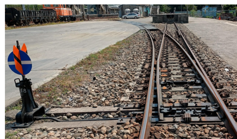
Image ⑥ The switch is placed on the left side Compared with image 5, the installation position of the switch is different for the 50 kg-N #8 articulated left switch
