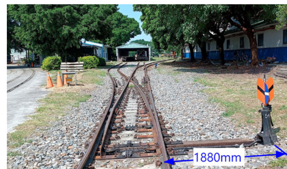
Image ③ Medium-sized marker-type switch The distance between the medium-sized marker-type switch and the gauge line is 1,880 mm
