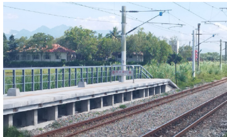
Platform elevation was completed at Sanmin Station
