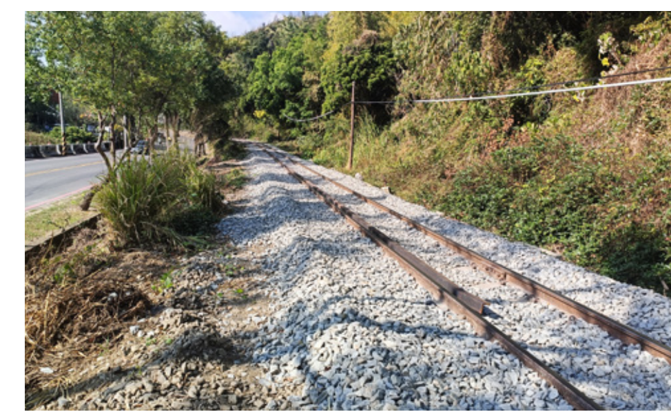
Track engineering (replacement of ballast)
