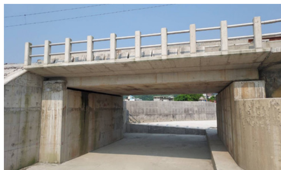
Xiaqijie Bridge reconstruction project (north side)
