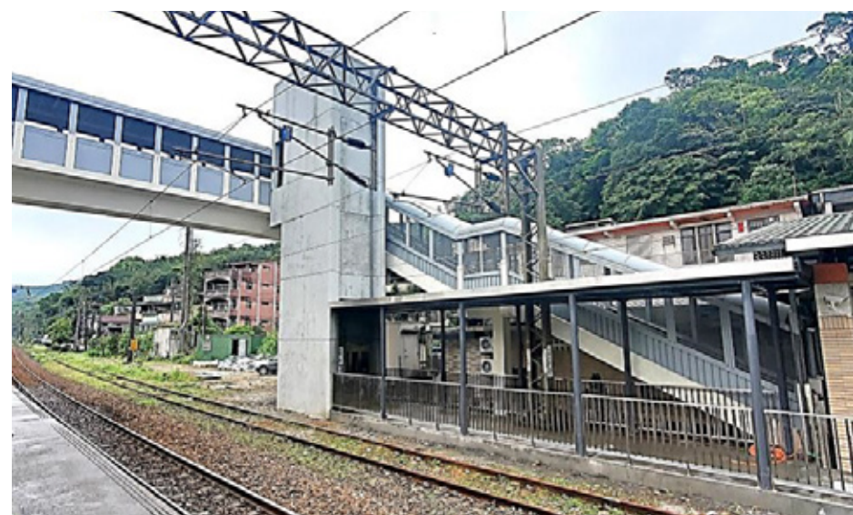
Newly installed barrier-free elevator at Gongliao Station
