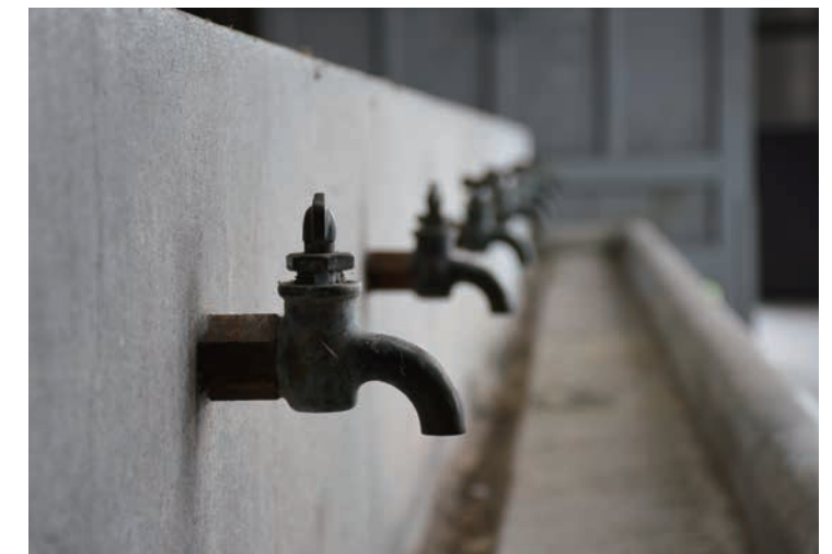
員工浴室中充滿古樸味的青銅製水龍頭，都是機廠員工自己翻砂打造的。它可以360度旋轉，只要開關和出水口呈90度就會自動止水，造型也比現代水龍頭厚重沈穩 The rustic bronze faucets in the employee's bathroom were cast by employees themselves. The faucets can be turned 360 degrees, and the water stops when it is turned 90 degrees from vertical. These faucets are sturdier than most of their modern counterparts.
