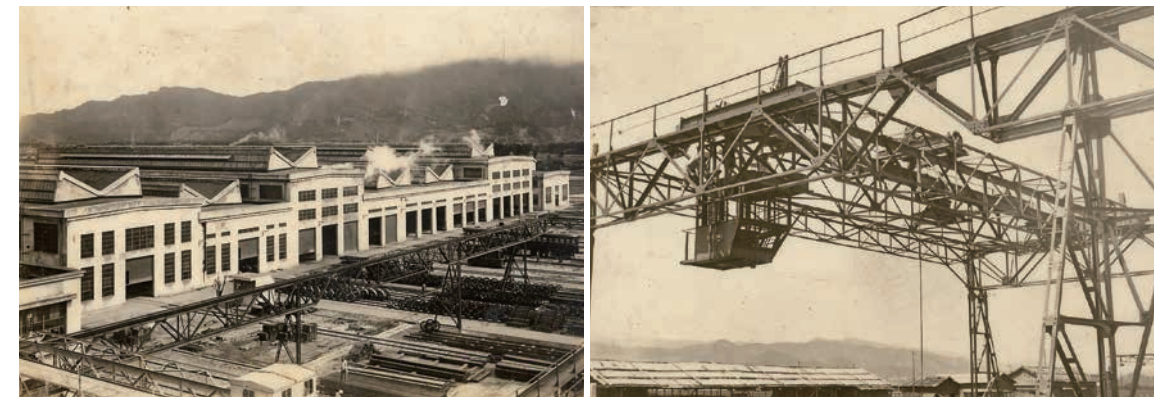
（左圖）油漆工場及移車台，維修好的車輛可直接由移車台送往工場油漆 （右圖）工場內的露天吊車，負責運送維修所需的原料 (Left) Repaired trains can proceed directly via the railyard to the Paint Shop. (Right) This overhead crane brought in all the materials needed to conduct repairs.
