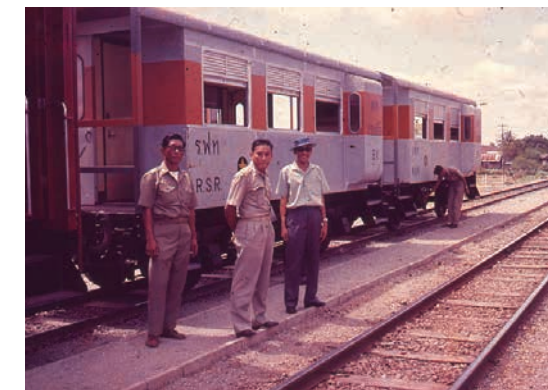
運抵泰國後進行試車 Cabooses undergo trial operations upon arriving.
