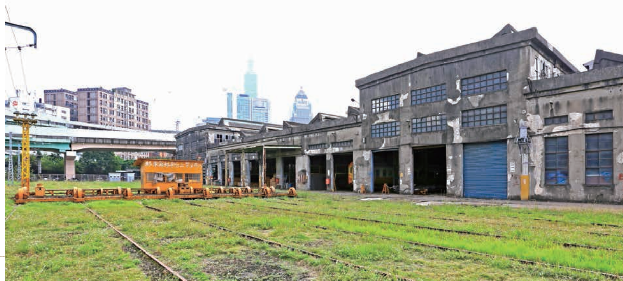
鋸齒型屋頂及移車台 The zig-zagged roof and the railyard.
