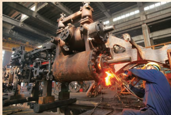
汽缸拆解 Removing the cylinder.
