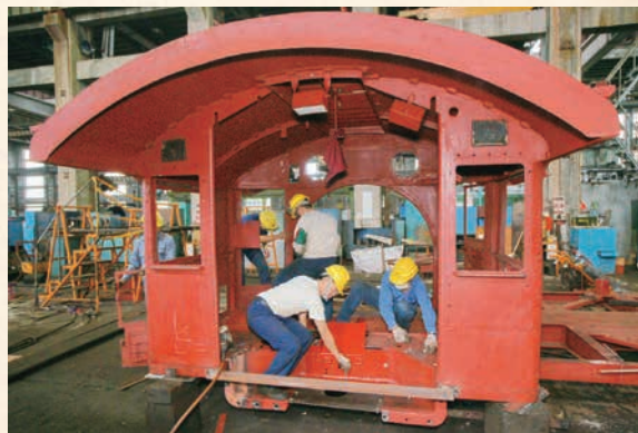
司機室整修 Restoring the driver's cabin.
