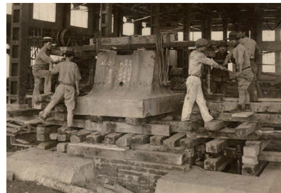
鍛冶工場蒸氣錘基座安裝 The base for the steam hammer is installed at the forge and metallurgy shop.
