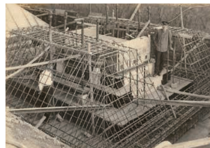
完成鋼筋作業的廠房基座 Rebar is being installed.
