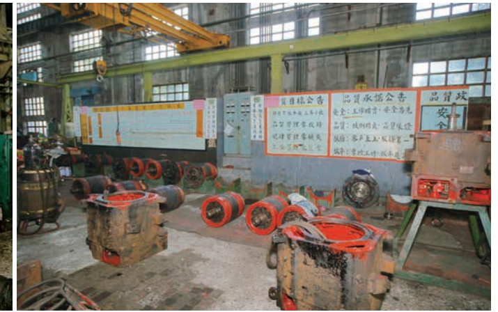
柴電工區電機二場看板上的馬達維修流程表 Motor repair at the diesel power workshop of No. 2 Electric Shop.
