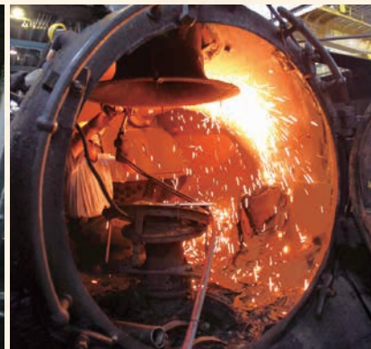
CT273 煙箱拆卸 Removing the CT273's smokebox.
