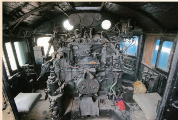
CT273 整修前 CT273 before restoration.
