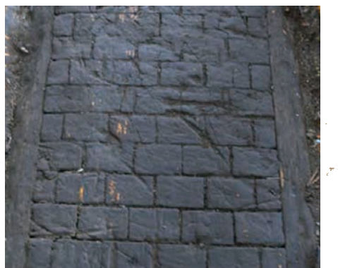
軟質木煉瓦地坪可避免維修零組件掉落地面造成損傷 Wooden tile floors can avoid damage components falling on the ground.
