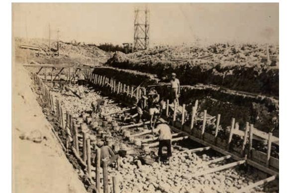
建廠初期，工人正在進行廠房基礎作業 Workers prepare the ground for the TRW's construction.
