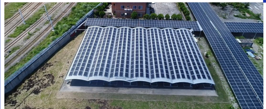
Solar photovoltaic power generation equipment installed on the rooftops of Taitung Station and its surrounding buildings, parking lot roof, and covered walkways
