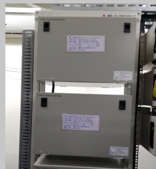
96-core optical fiber cable control room
