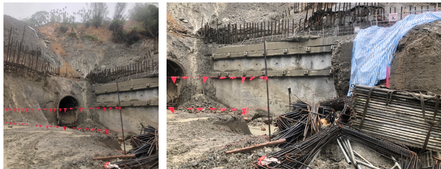
Chiayi Construction Branch cut-and-cover tunnel construction on the Jiji Line
