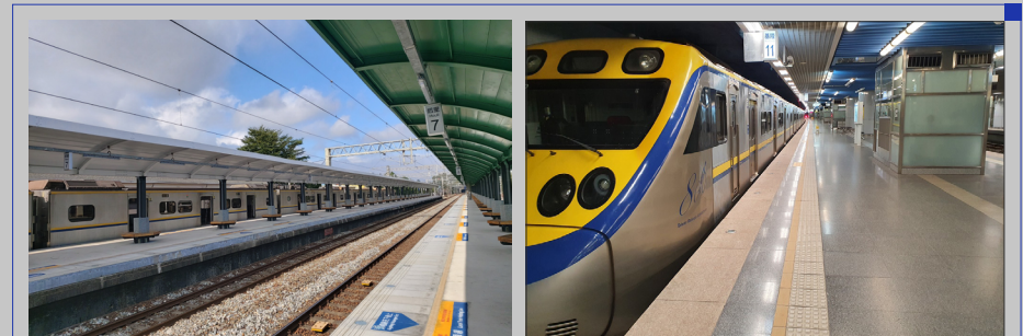
Increased platform height at Houli Station
