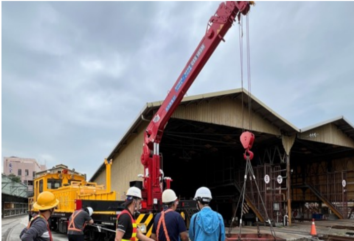
Load-bearing test of the boom on railway mobile crane cars
