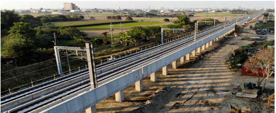
Wencuobu Creek Bridge Reconstruction Project (Aerial View)
