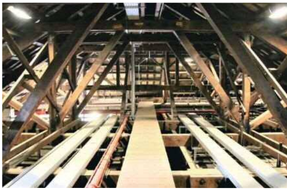
▲屋頂木製桁架樑柱
