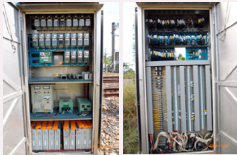
Large safety relay-type control unit after replacement
