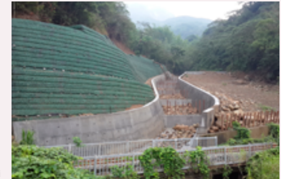
Slope failure recovery project in Jiji
