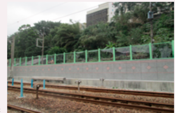
Ruifang acoustical barrier project
