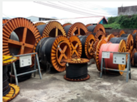
Outdoor material stored in areas and installed with a signboard(2)
