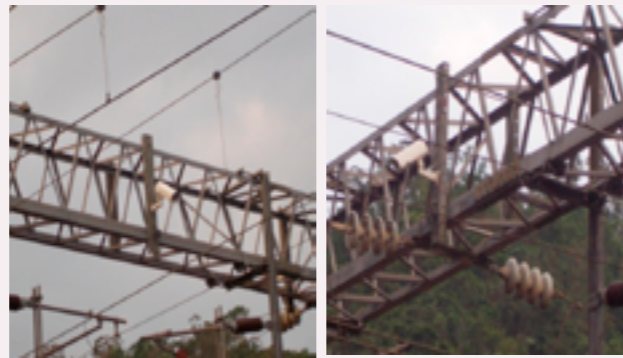
Set up monitoring devices
