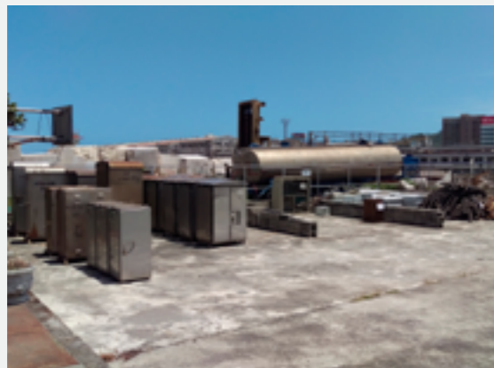
Outdoor material stored in areas and installed with a signboard(1)
