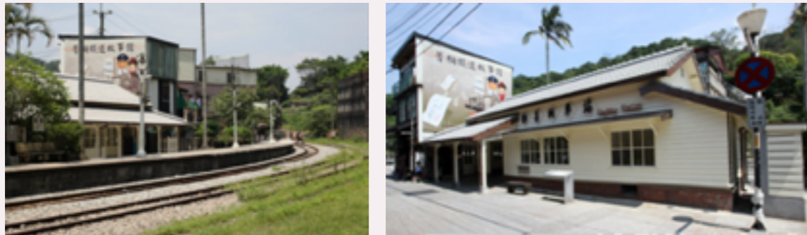
Jingtong station relic recovery project
