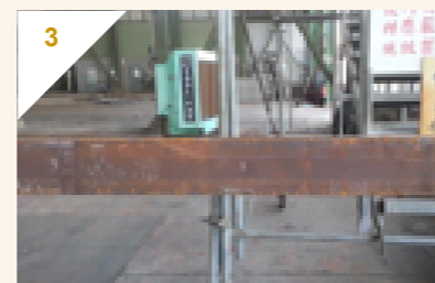
3 Mark the processing area at the bottom
