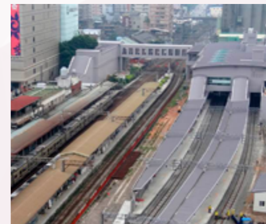
View of the temporary station in Taoyuan
