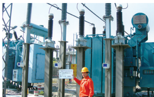
● 變壓器容量擴充(左15MVA，右25MVA) Expansion of transformer capacity to (left 15MVA, right 25MVA)
