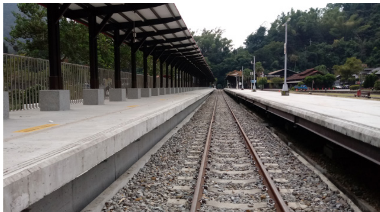
Platform addition and track strength enhancement project of Checheng Station
