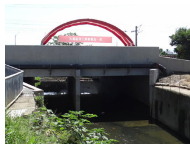
Completed First Minxiong bridge
