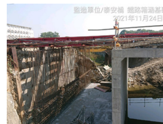
Construction of new box culverts of Tai'an Bridge
