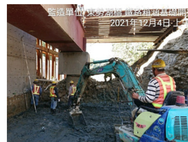
Construction of new box culverts of Dongshihu Bridge
