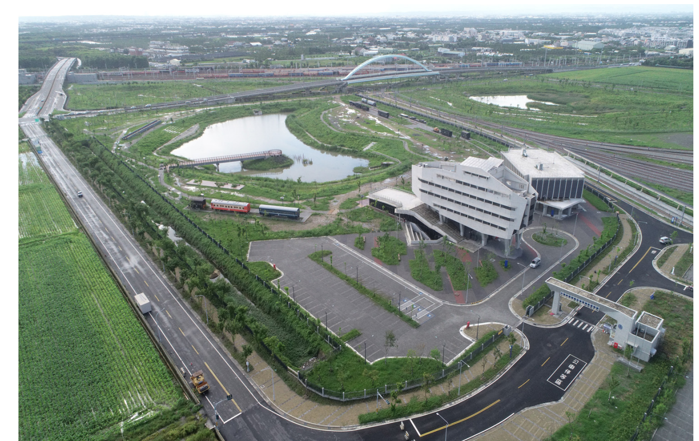
Aerial Photos of Kaohsiung Workshop and Chaozhou Depot
