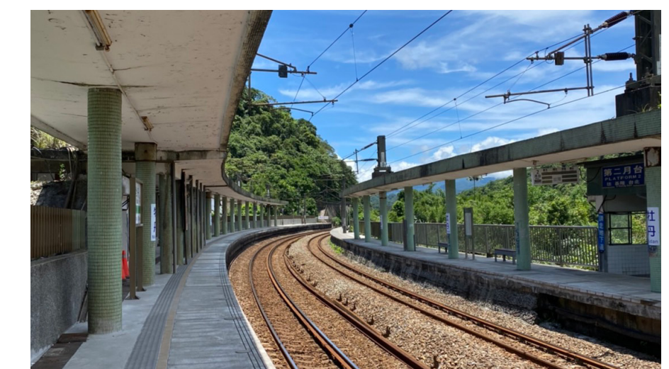
Completed platform raising project of Mudan Station
