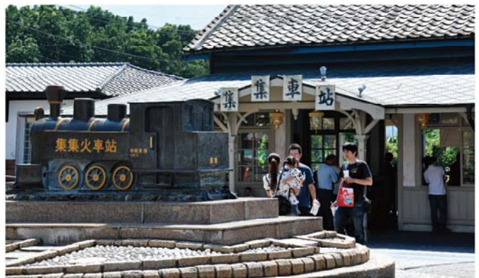
921 大地震造成集集火車站嚴重損毀，幾經重建之後，如今重回繁華景象。 Jiji Station was severely damaged by 921 earthquake, but now has regained its prosperity after several reconstructions.
