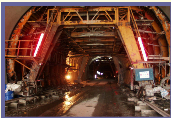
(4)滑動模組內襯砌施工
